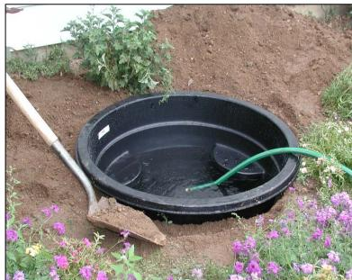
Bed the pond on a layer of sand, then level. Once the pond is leveled, backfill with loose dirt between pond and excavation, stopping at the halfway mark between excavation base and pond's flange.
